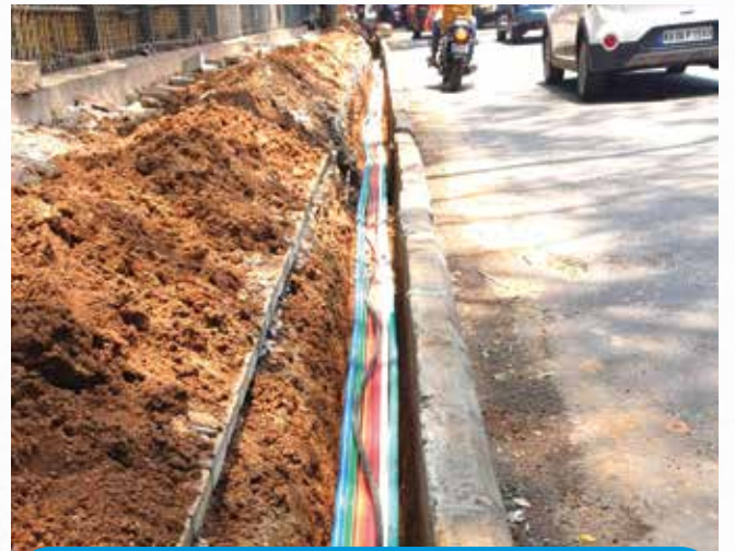
OFC cables laid underground in all arterial & sub-arterial roads
