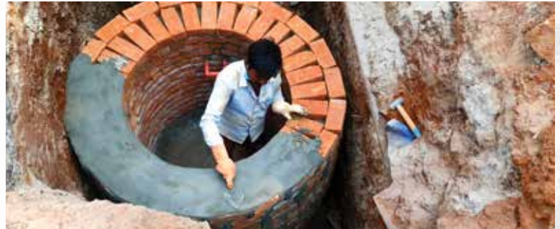
All UGDs & manholes being rehauled to eliminate sinkholes
