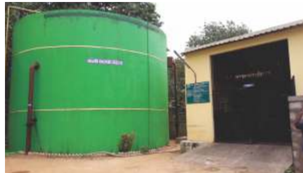
Bio Methanation Plant, MSR Road, Subedar Palya.
